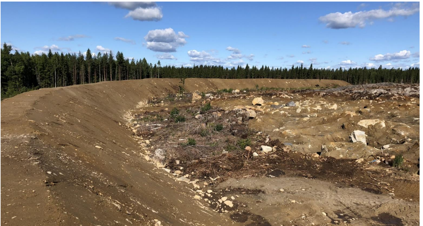
Figure 3 – Construction of noise barrier at the Kaapelinkulma Gold Mine.
